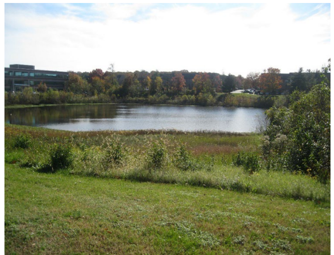
Figure 6 - Existing stormwater management pond along the east side of Hanover Parkway
