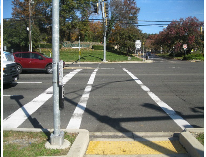
Figure 4 - Crosswalk approach on the west leg of MD 193 (Greenbelt Road) at Hanover Parkway
