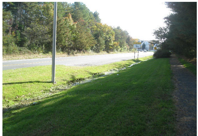
Figure 8 - Existing roadside ditch along Hanover Parkway, south of traffic circle
