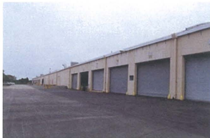
GSA Franconia Warehouse Complex - Building A
