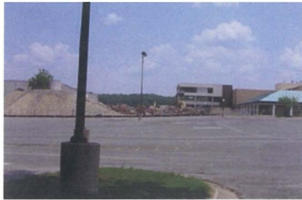
Landover Mall during Demolition (2006).
