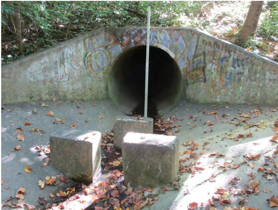
60-1. 09/28/2017: Outfall 60, facing southeast. Looking at the outfall.
