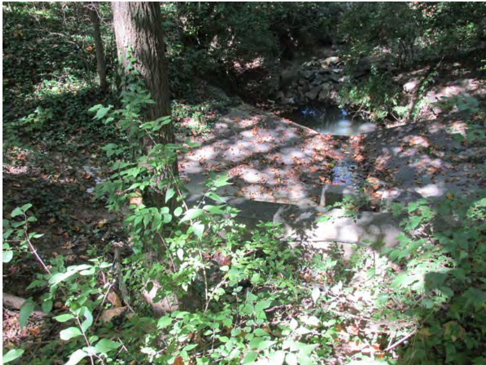
60-4. 09/28/2017: Outfall 60, facing northwest. Looking downstream.
