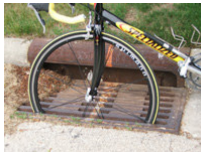
Bicycle wheel in drain grate
