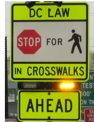
Rapid flashing beacon
