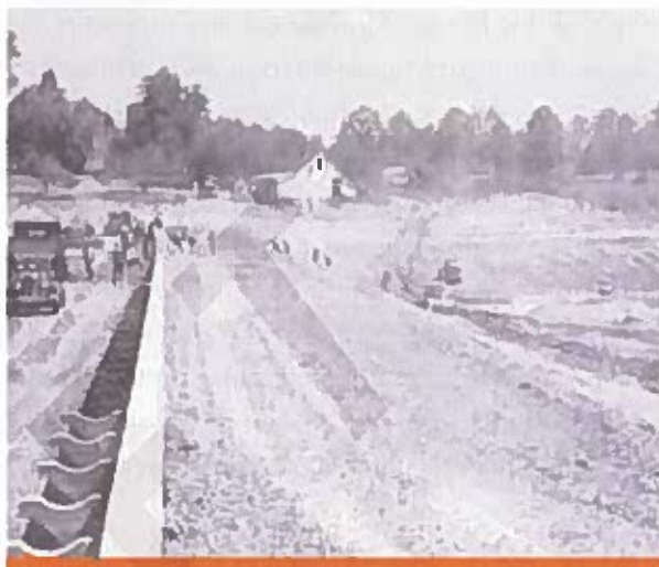
FIGURE 9 Dam construction at Greenbelt Lake.
