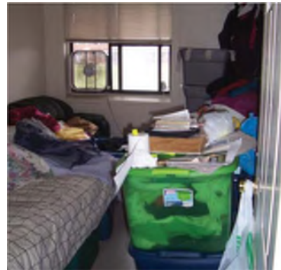
Life Safety: No A/C within units; window-mounted fan doesn't permit emergency access through only bedroom window.
