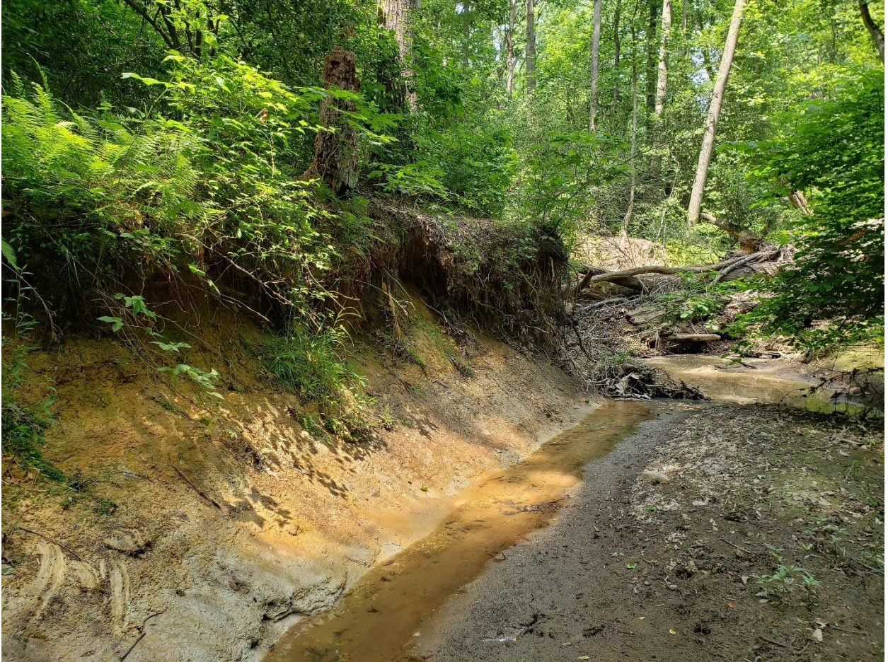
Figure 1. Under cut trail and partial dam along Goddard Branch Trail in the North Woods Tract
