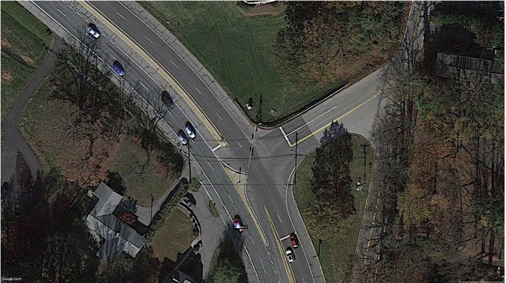
PHOTO OF EXISTING MARYLAND “T” INTERSECTION
