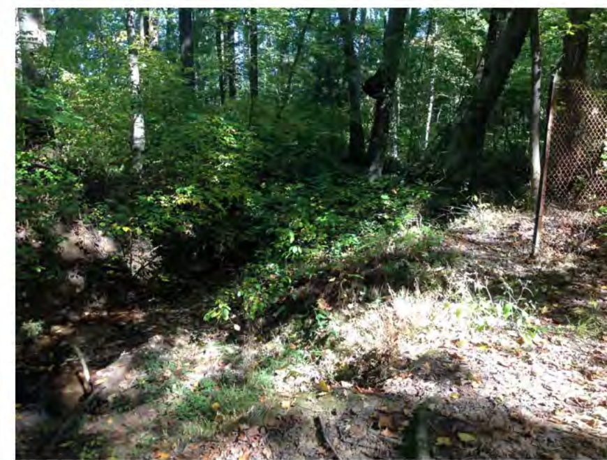
C - Broken fence atop Beaverdam Creek tributary
