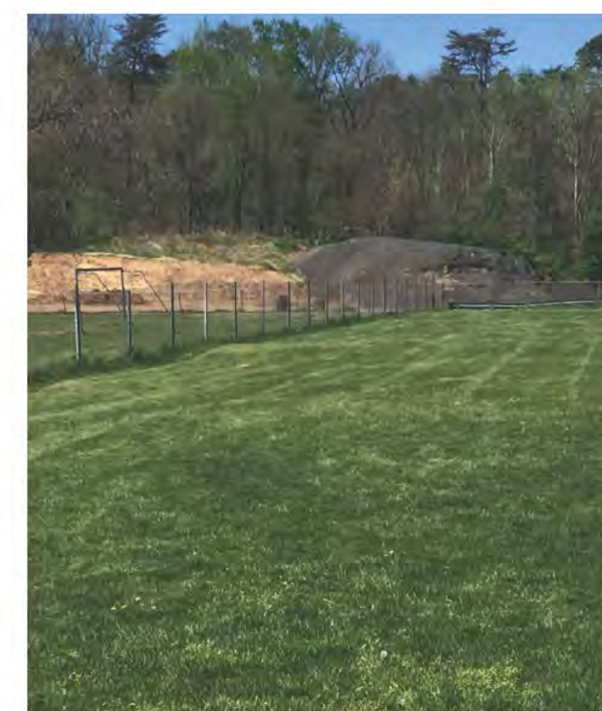
D - Stockpiles for asphalt millings and soil encroach into the forest.
