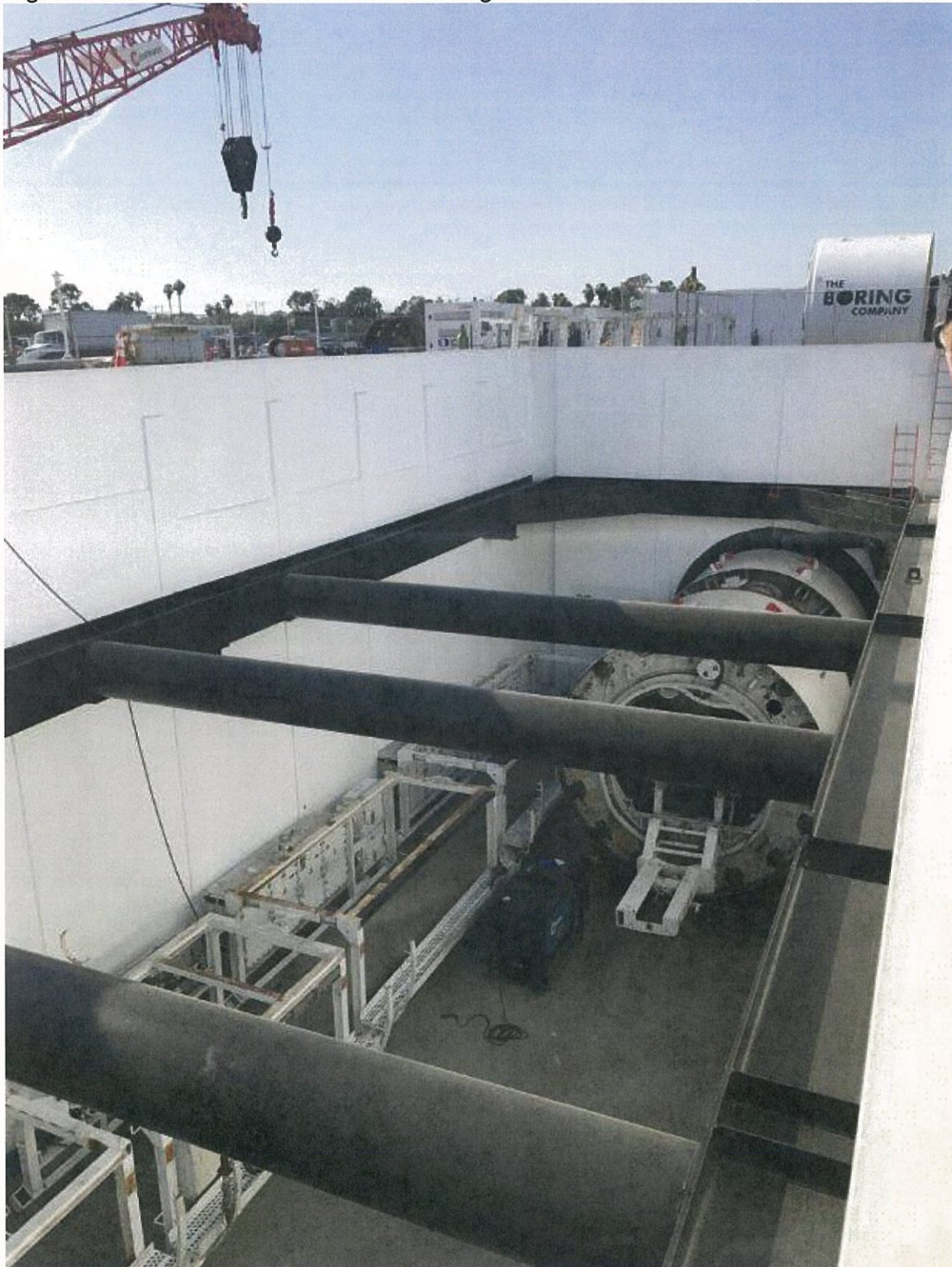
Figure 2: TBM Launch Shaft at the testing location in Hawthorne, CA 2
