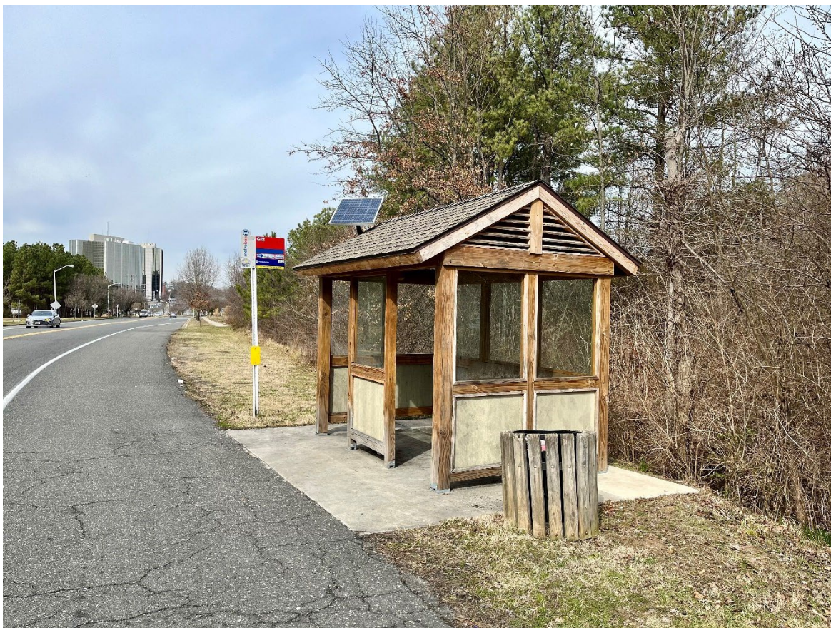
Figure 4 – Solar powered lighting on a bus stop shelter
