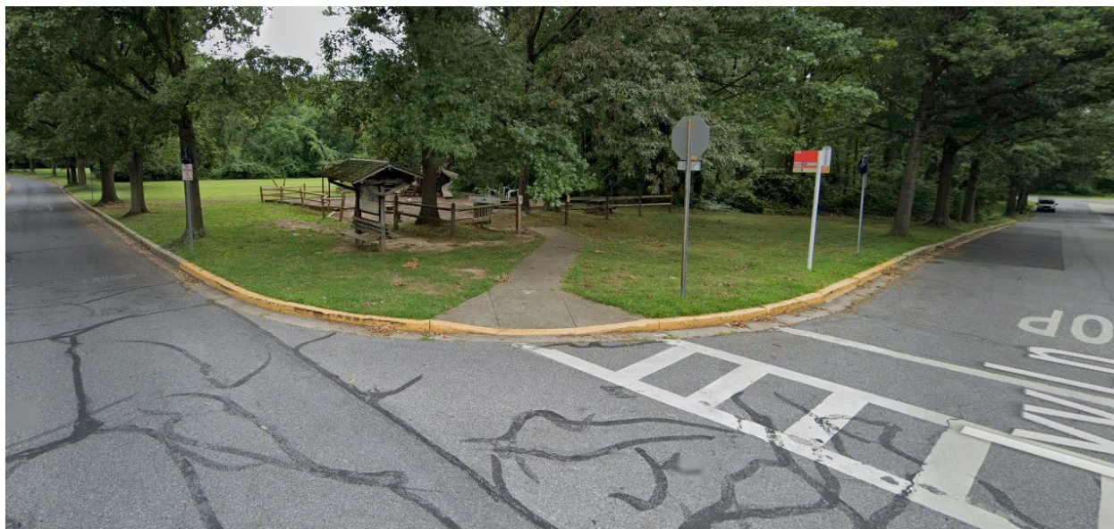
Figure 1 – Example of a bus stop in need of a short sidewalk extension and landing pad for access
