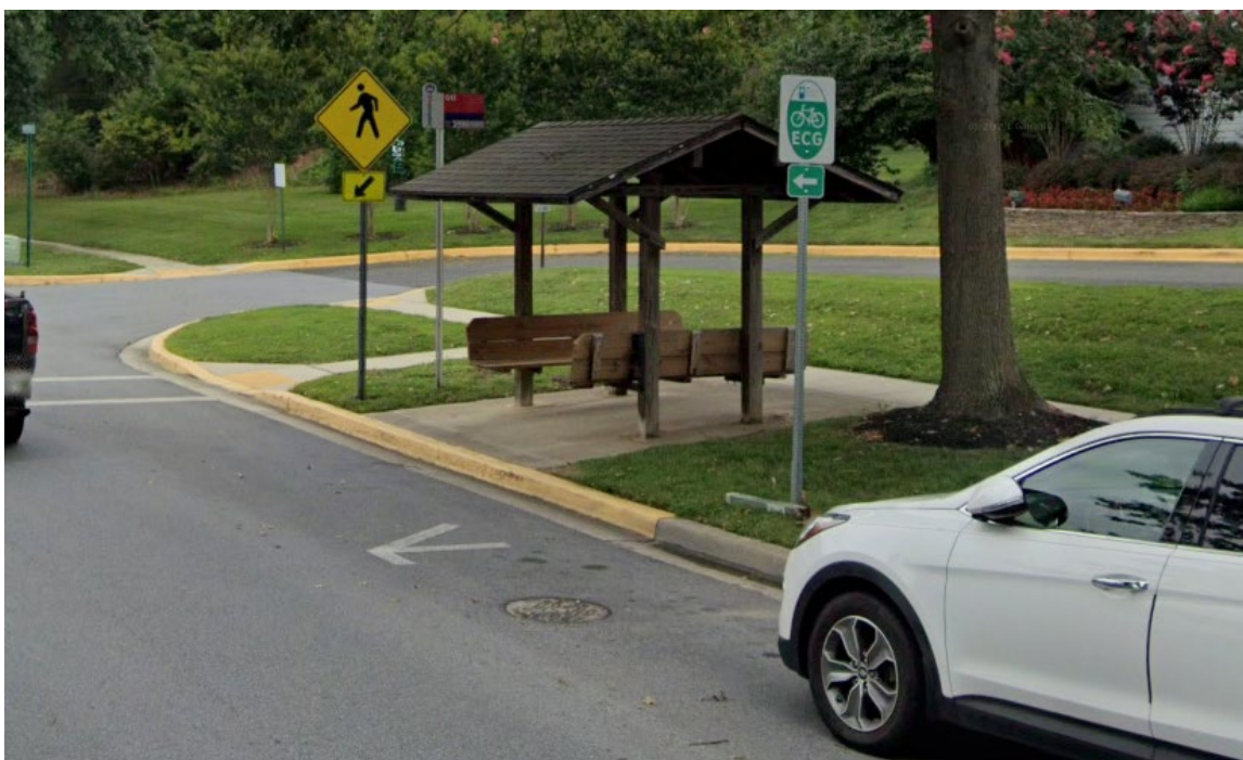
Figure 5 – Example of a shelter that blocks ADA access
