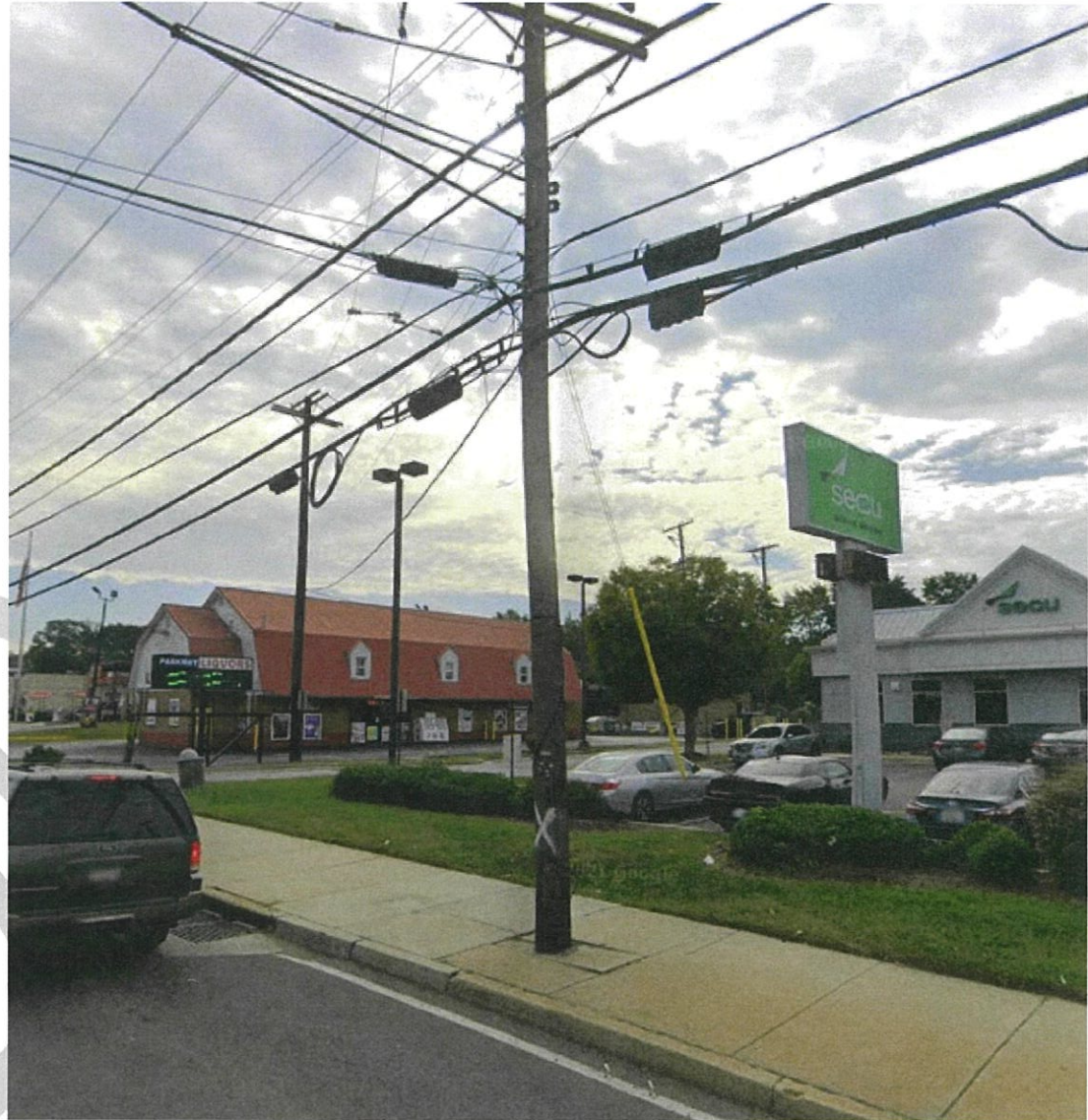
Figure 18. Utility pole in the middle of the sidewalk between Cunningham Drive and 61 st Avenue (Google Streetview)
