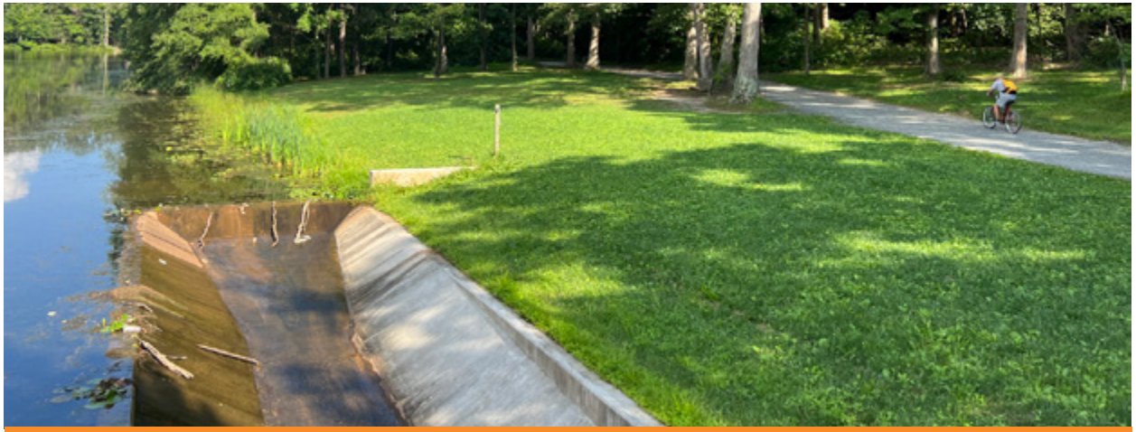
FIGURE 6 Site photos of existing conditions at Buddy Attick Park.
