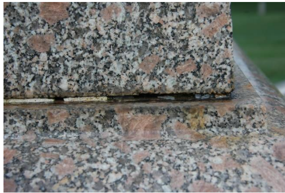
failing joints
