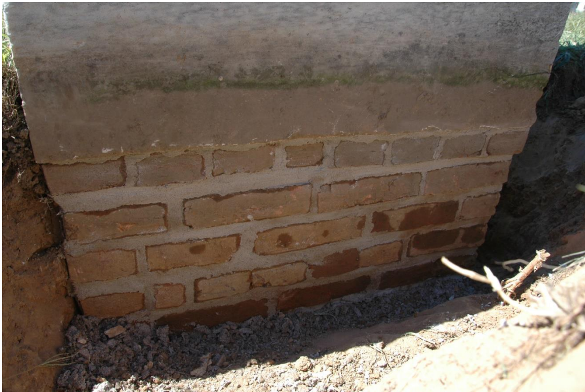
East wall, after repointing.
