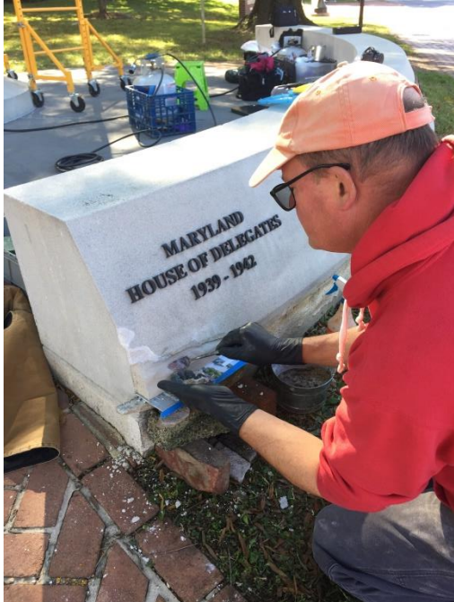
Goldstein Memorial during treatment.
