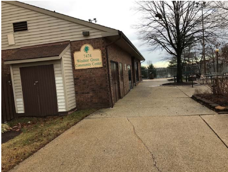
CLOSE UP VIEW BUILDING PLAZA IS TO THE RIGHT
