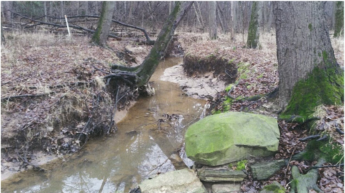
View upstream along Reach 3, stream channel along this reach is narrow and slightly more incised than Reach 4.
