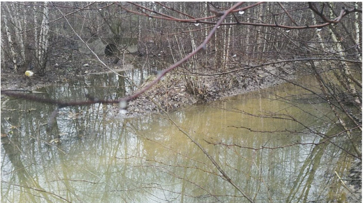
Storm drain outfall into Reach 4 at stream outfall into the pond.
