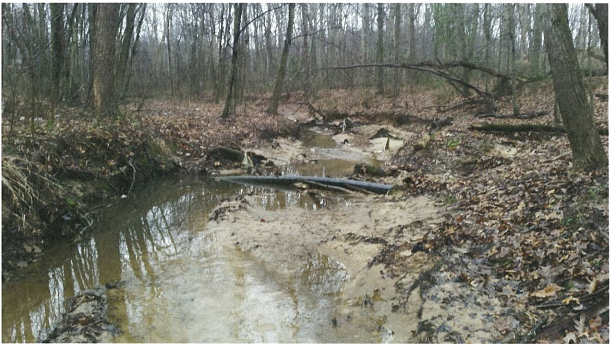
View upstream along Reach 2 of exposed possible sewer/water line crossing in the stream channel.
