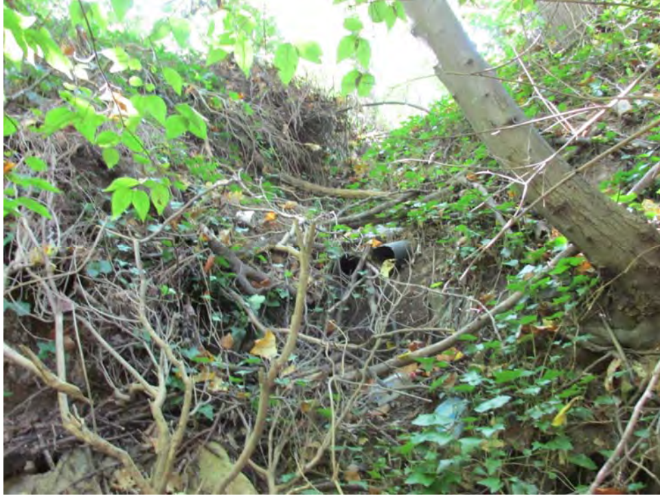
60-3. 09/28/2017: Outfall 60, facing southwest. Looking at stormwater drainage pipes.
