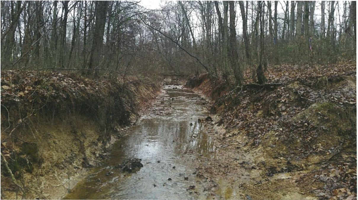
View upstream along Reach 1. In this section of the reach the stream channel narrows and is more of a box cut into the hard clay. The banks are a mixture of sand and clay and actively eroding.
