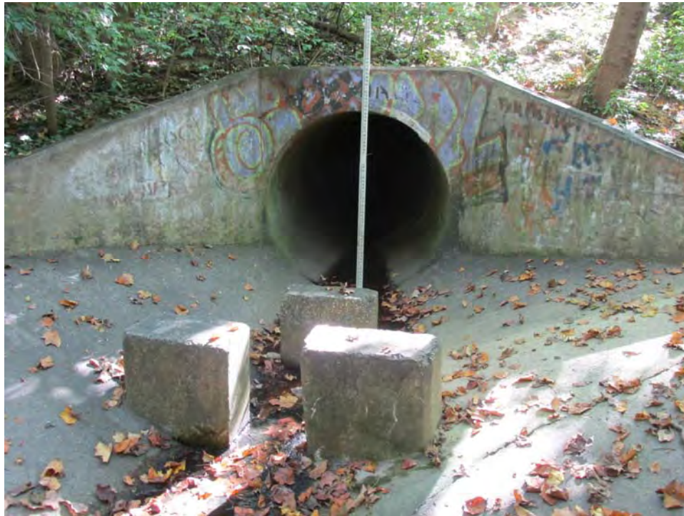
60-1. 09/28/2017: Outfall 60, facing southeast. Looking at the outfall.
