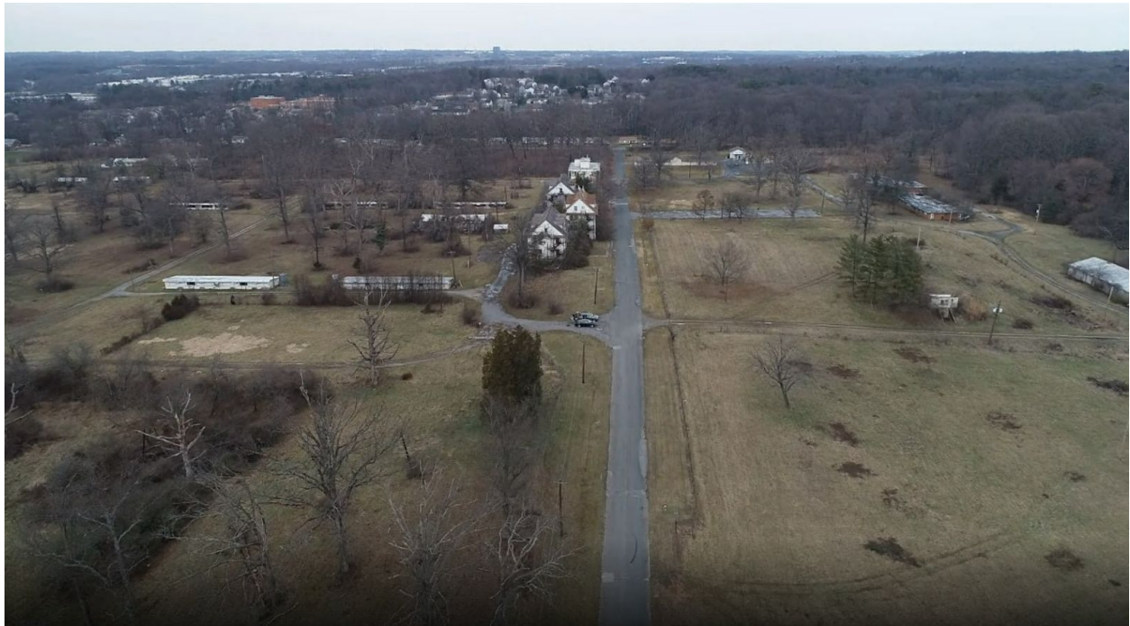
Aerial view along Poultry Road looking north
