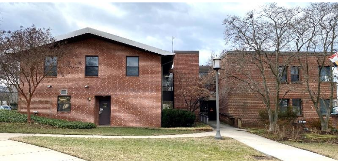
From Crescent Rd & Southway
