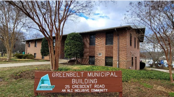
From Crescent Rd & South Dr. – 1964 Wing
