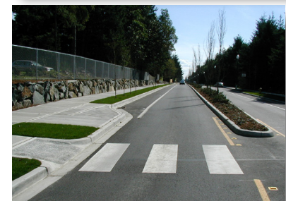
Options for improving crosswalk safety include refuge islands and striped or raised crosswalks.
