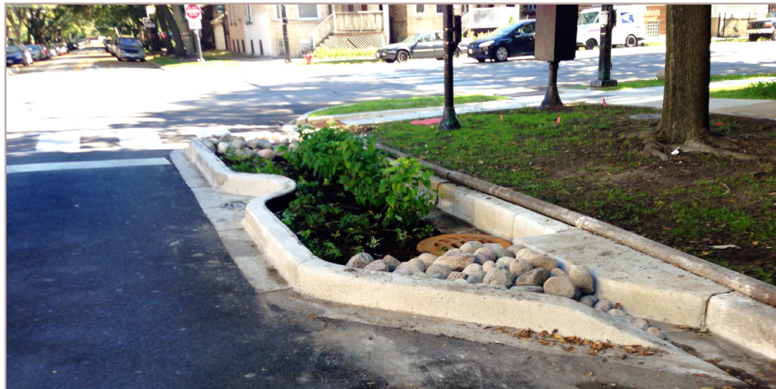
Example of a stormwater curb extension along side a residential street.
