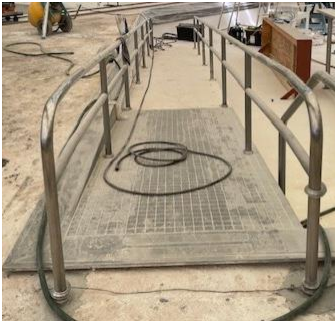
Indoor Pool Ramp with Handrails
