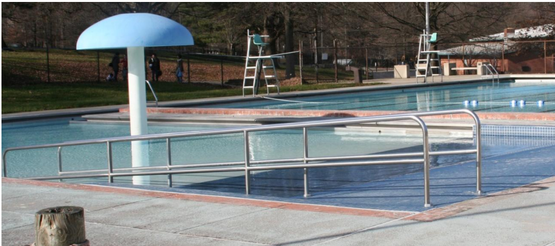
Outdoor Pool Ramp with Handrails and Zero Depth Entry
