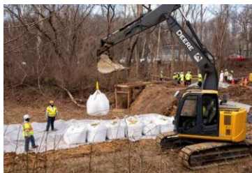
Workers build a cofferdam to stop the flow of raw sewage into the Potomac River after a massive sewage pipe rupture in Glen Echo on Jan. 23. (Cliff Owen/AP)
