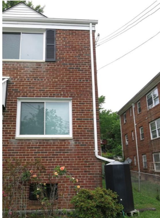
Figure 28: Examples of rain barrels. (photos courtesy of DOEE website https://www.riversmarthomes.org/gallery )
