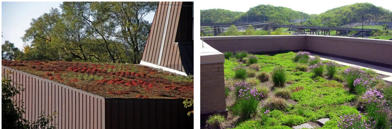
Figure 25: Examples of green roofs (photos courtesy of LimnoTech)
