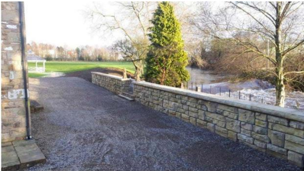
Figure 21: Example of a flood wall installed between a building and a river (Image courtesy of Redi Rocks website: redi-rock.com)
