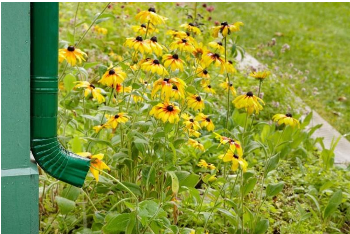
Figure 27: Examples of rooftop disconnection to a pervious surface. (photos courtesy of EPA: https://www.epa.gov/green-infrastructure/types-green-infrastructure )
