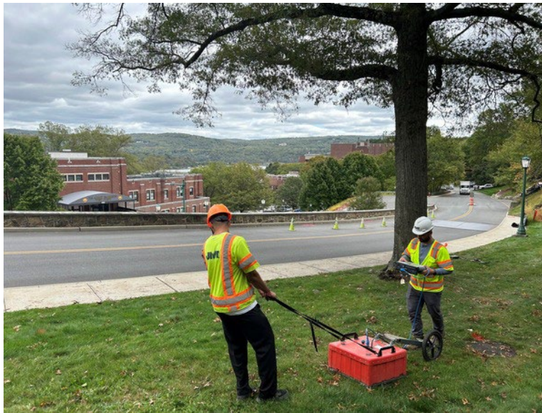
Photograph 35. An example photo of GPR equipment being used by workers to locate subsurface utilities.
